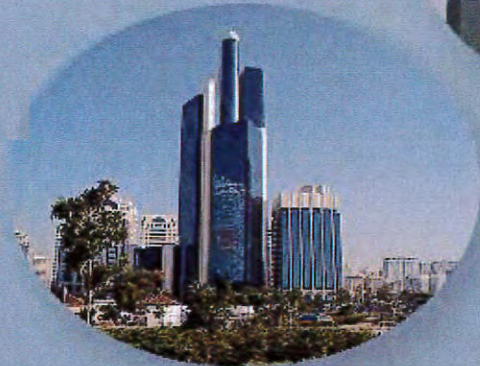
Baynounah Hotel In-Building GSM Coverage
