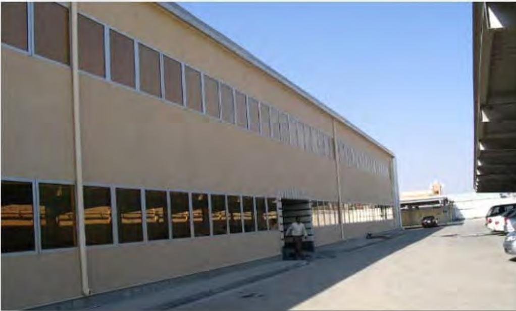
Our datacenter from outside
