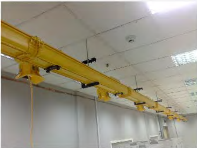
Optical Fiber Cable Tray and accessories
