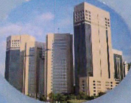
Sheikh Khalifa Energy Complex In-Building GSM Coverage
