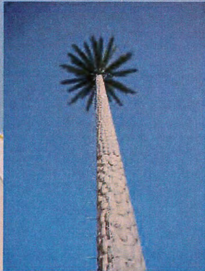
Camouflage Communication Tower One of many others built in VIP areas
